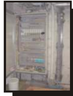
new shore connection HV room to accommodate the new HV circuit breaker cubicle
