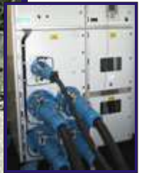
Patton and Cooke C150 Series Plugs and Receptacles mounted on an ABB power management System
